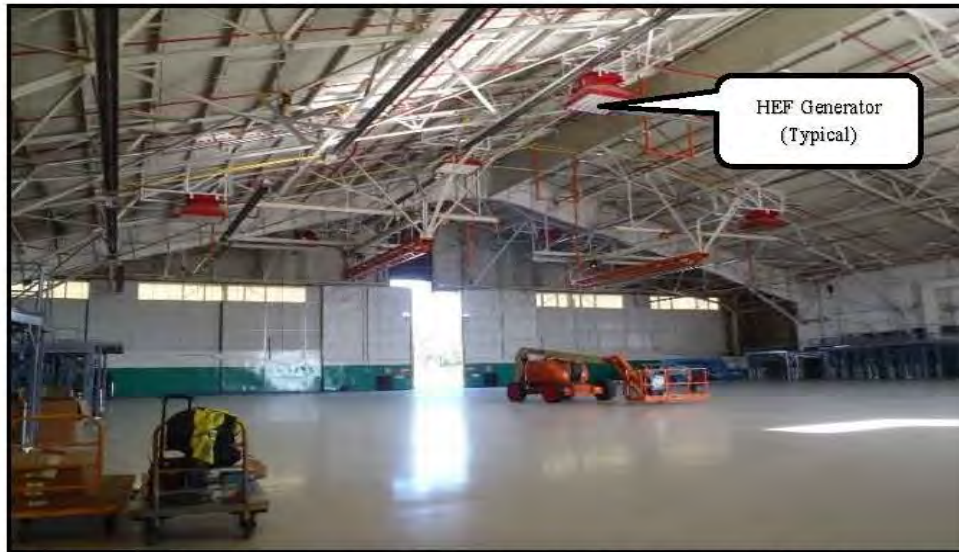
Photograph 3: Building 1905, view looking northwest (interior) of installed HEF Generators.
